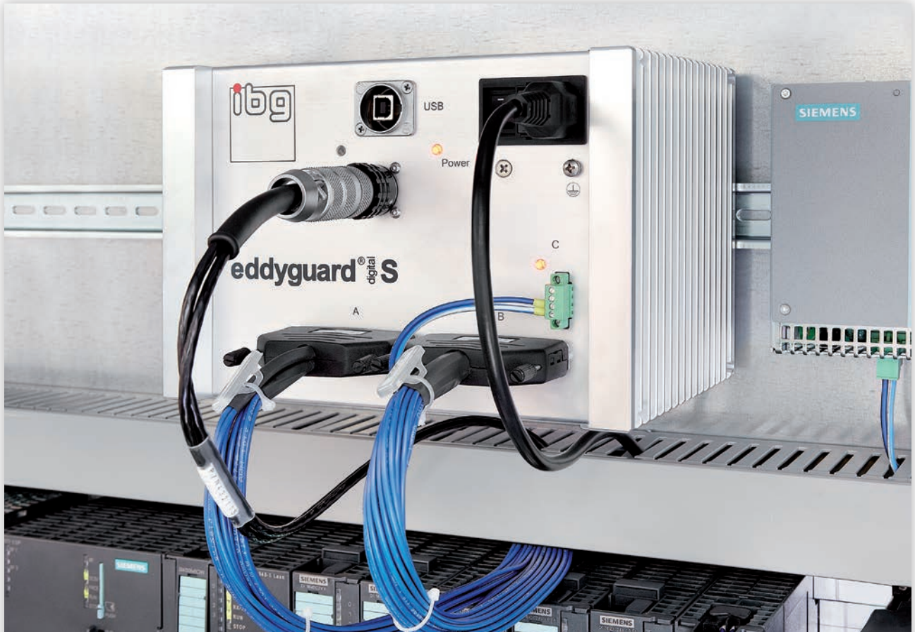
Designed for the switching cabinet: eddyguard S in built-in situation.
