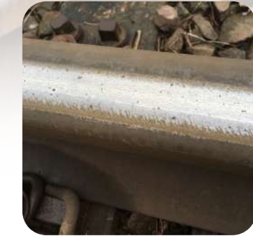
Detected Defects on Rail
